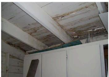
∨ The roof rafters are minimally supported by a rotated ridge board. Further evaluation and additional support are recommended.
