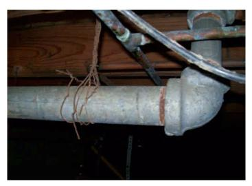
There are exposed water pipes running through unheated space, which should be insulated to guard against energy loss, freezing, and damage to the piping and dwelling.
