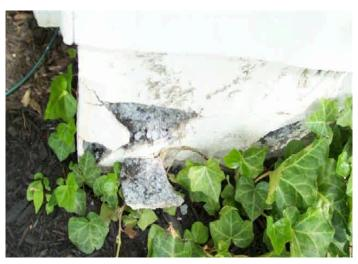
Several of the crawlspace vents are at soil grade level has allowed moisture and related conditions (deterioration/rot and WDI infestation, etc.). As an upgrade, installation of the "well or wells" is recommended. Consult with an qualified contractor for details and estimates.
