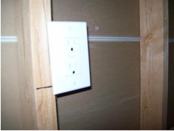
Location Room: Basement Equipment: GFCI Outlet
