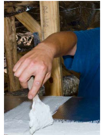
Above: Paint mastic (a thick, gooey substance) onto the duct seams and joints. (Photo source: Habitat for Humanity, Lakeland, FL)
