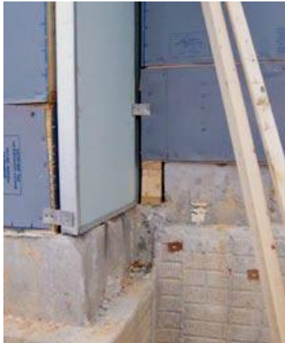
Above: Seal air gaps between two framed common walls. (Source: Energy Services Group via the EPA, 2008)
